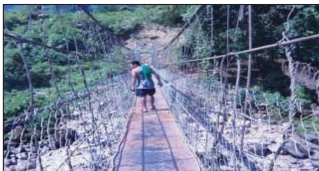
Construction of Reinforced Cement Concrete (RCC) Pillar Wire Rope Suspension Bridge (WRSB) over Kumey river in between Mangio village to Government inter village school Pachangriang Mangio, Block Parsi Parlo, District: Kurung Kumey (Arunachal Pradesh) under (BADP)
