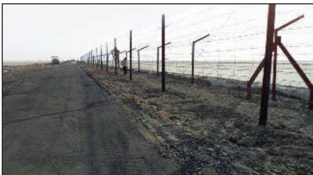
Pilot project along the Gujarat Border.
