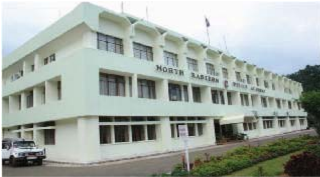
NEPA Administrative Building
