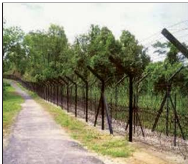
Fencing and Road along IBB
