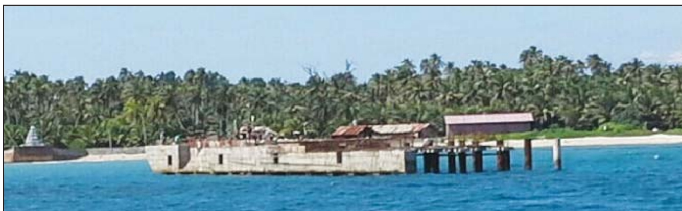
Re-Construction of Jetty at Teresa for berthing of speed boats
