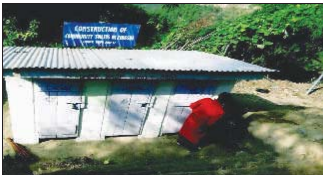
Construction of Community Toilets at Zingsui District: Ukhrul (Manipur) under BADP
