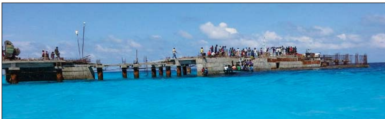
Re-Construction of (Marine Hard) Jetty at Chowra.
