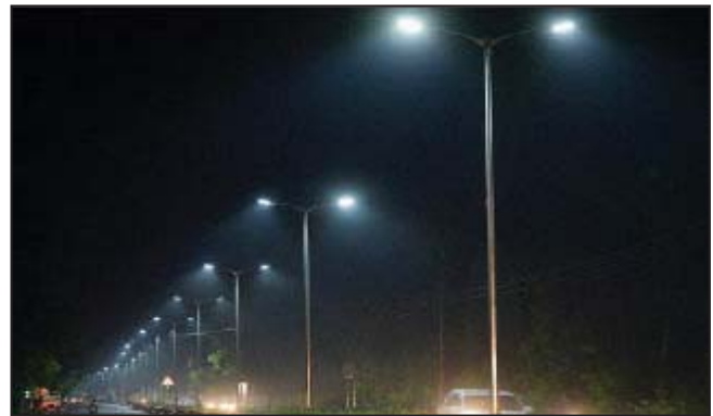
A view of LED Street Lights
