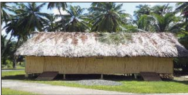
View of the Eco-friendly Cycle Stand constructed with locally available materials under MGNREGA in convergence with PYKKA at Perka Village, Car Nicobar, Nicobar District.
