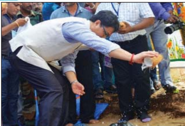
Shri Kiren Rijju, Minister of State (Home Affairs) Laying Foundation Stone of Tad Bridge at Tad Creek at Diu
