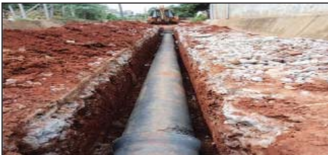
Sewer line works
