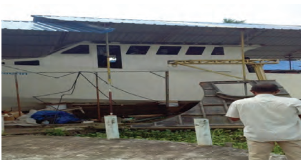
65" FRP multi day fishing vessel under construction for Fisheries Department
