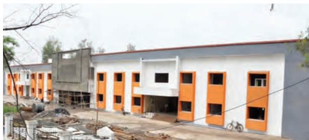
Construction of Farmers Training Centre at Silvassa
