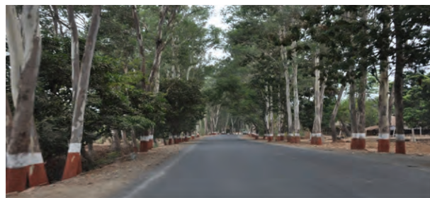
Construction of 4 - Lane Road from Kilwani Chowk to Silly Fatak
