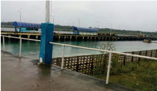
Extension of Jetty at Havelock
