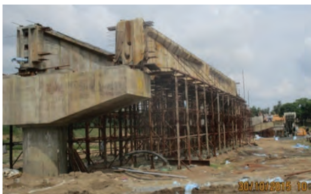
Construction of High Level bridge across Sankaraparani River - work in progress
