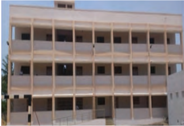
Government Higher Secondary School at Kirumampakkam
