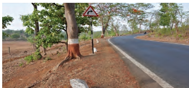
Widening of Khanvel - Khedpa road (Phase-II). (12.00 KM)
