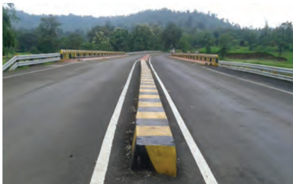
Construction of High level bridge at Karchond (4-lane bridge)
