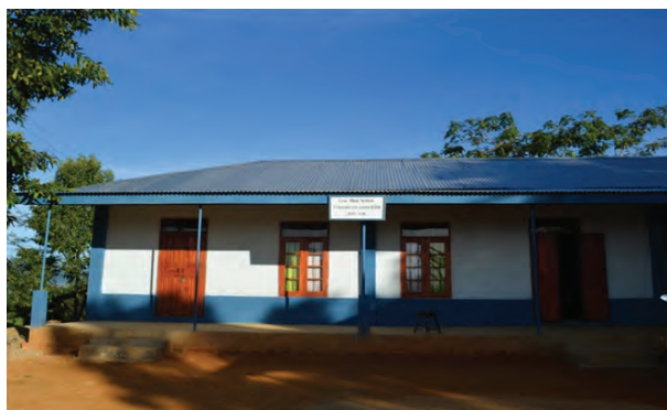
Construction of School Building at Leng, District: Serchhip (Mizoram) under BADP SCA: 2014-15.
