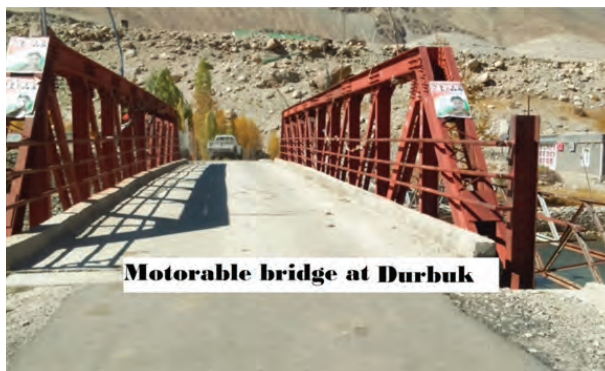
Construction of Motorable Bridge at Durbuk , District: District Leh (J&K) under BADP, SCA:- 2014-15
