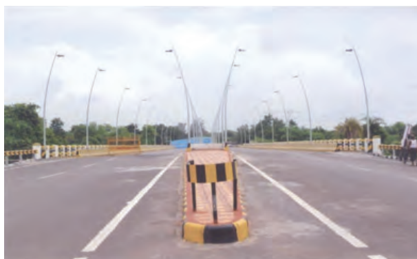
Construction of High Level Agriwad Bridge
