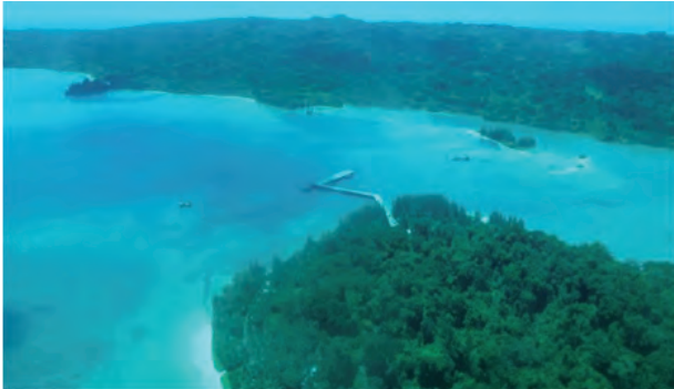
Construction of Jetty at Katchal
