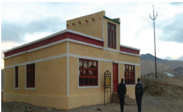
Construction of Public Health Centre at Chushul District: Leh (J&K) under BADP, SCA:- 2014-15
