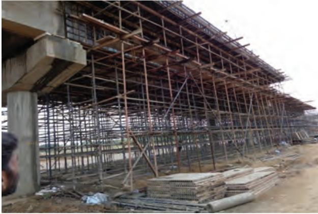
High Level Bridge across Sankaraparani river, Puducherry - Work in progress
