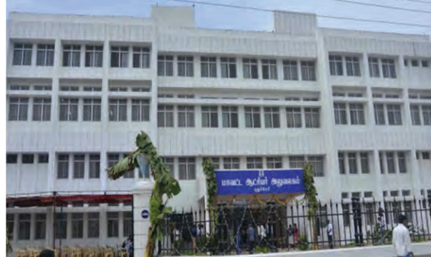
New Collectorate Building
