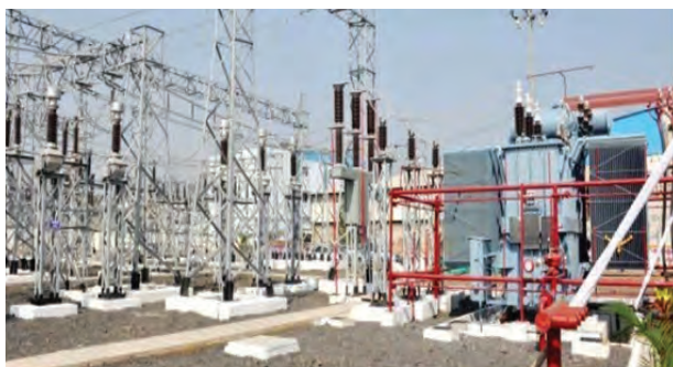
66/11 KV Substation, Kala started on 16/02/2015
