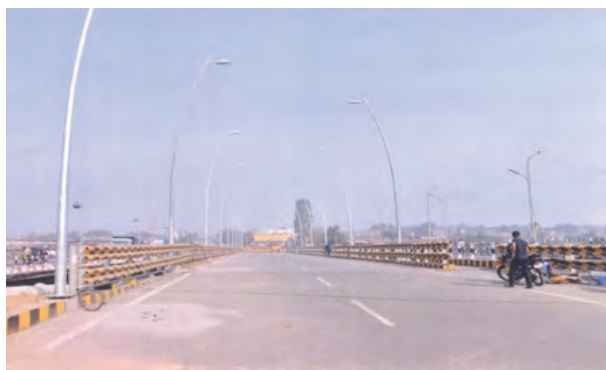
Construction of High Level Bridge at Piparia
