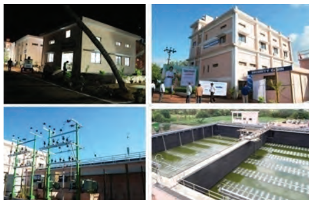
Sewerage Treatment Plant at Lawspet, Puducherry
