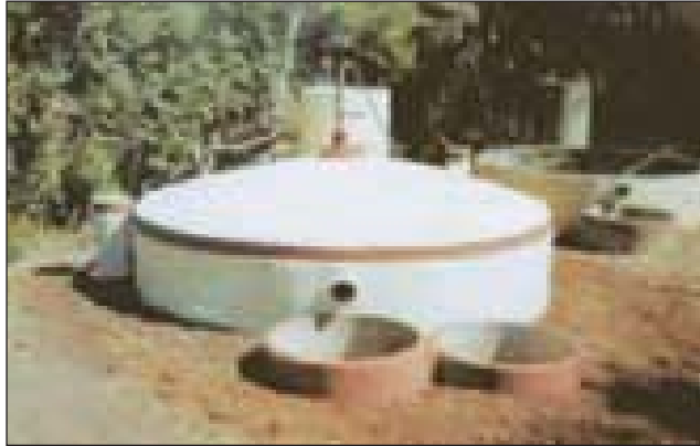
Setting up of Biogas Plant for management of Biodegradable waste
