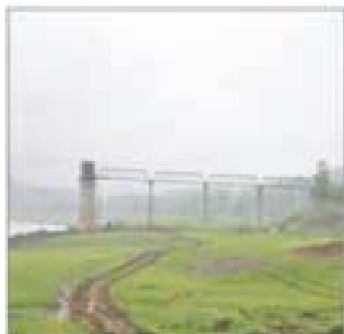
Water Supply Project for Dudhani & Mandori Patelad
