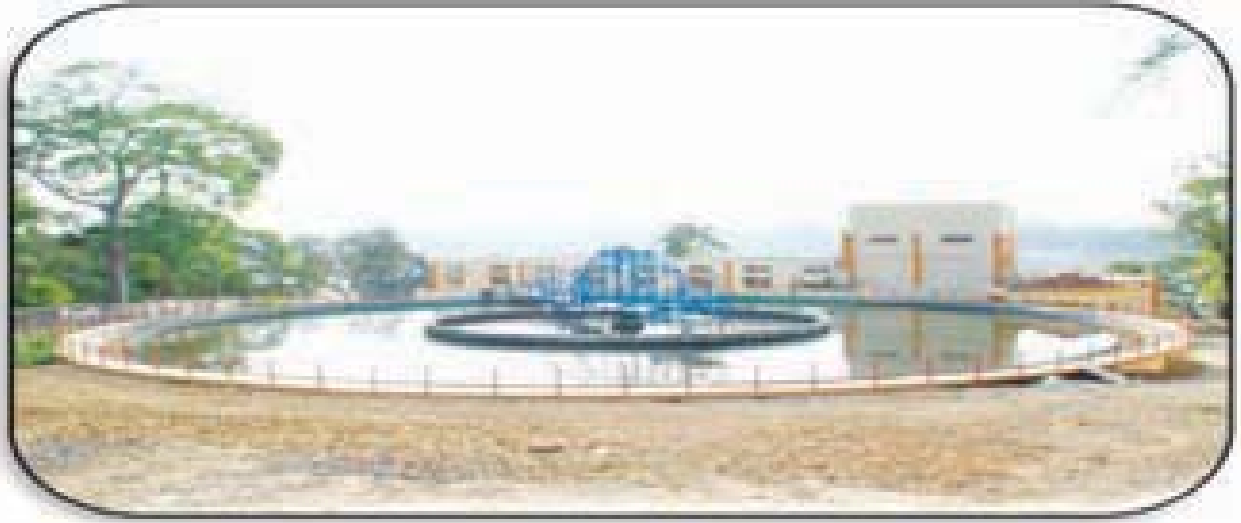
MLD treatment plant at Lambaline
