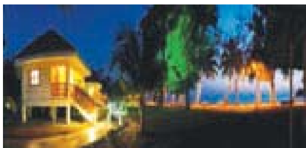
Refurbishment of Dolphin Resort Havelock
