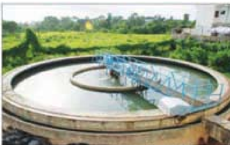
Water Supply Project for Silvassa Municipal Area
