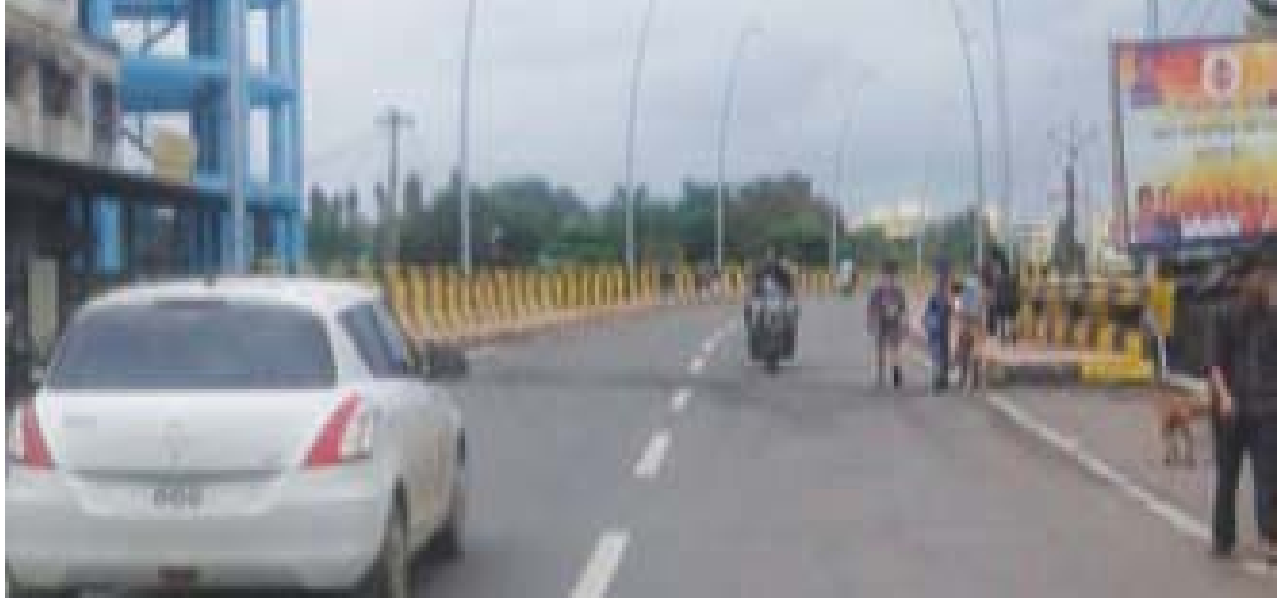
High level Bridge at Dokmardi
