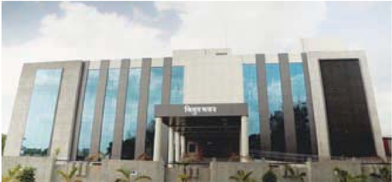
Construction of new office building of Power Department / DNHPDCL With estimated Cost of ₹21.00 crore has been completed and inaugurated.
