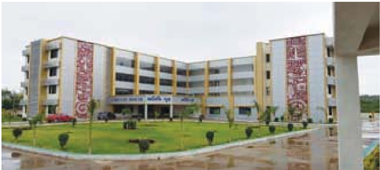
Construction of Circuit house at Silvassa with estimated cost of ₹16.50 crore has been completed.
