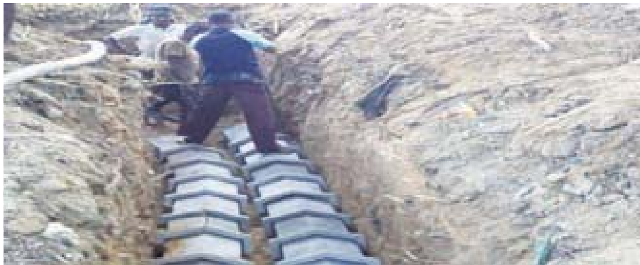
Laying of 11KV Underground cable with protective covering in the trench at Karaikal
