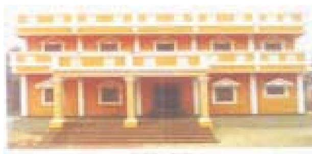
View of Community Hall at Kalmedupet, Puducherry
