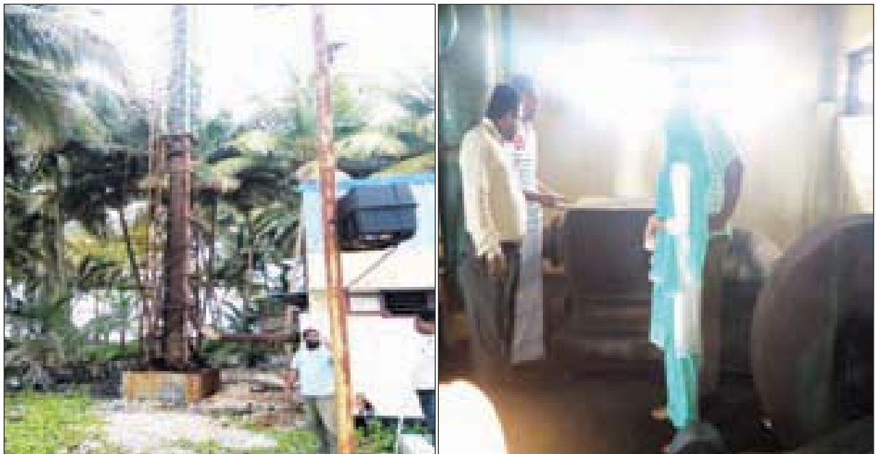
Installation of Incinerators
