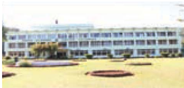
Administrative Building, NEPA
