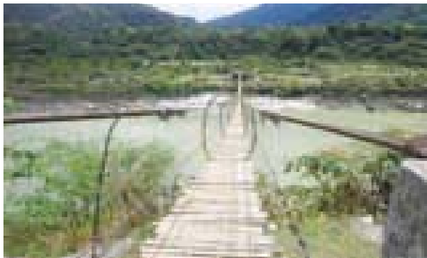
Construction of Foot Suspension Bridge over at Ladum point Tuting (Distt: Upper Siang), Arunachal Pradesh under BADP, SCA: 2014-15
