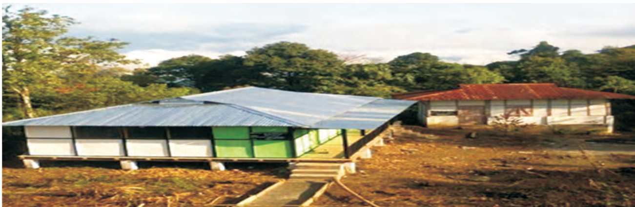
Construction of Community Hall at Migging-II village District: Upper Siang (Arunachal Pradesh): 2015-16
