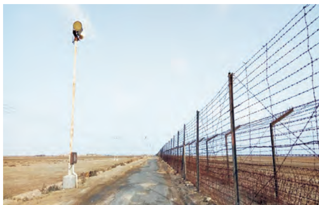
Fence & Floodlighting along Indo-Pakistan Border
