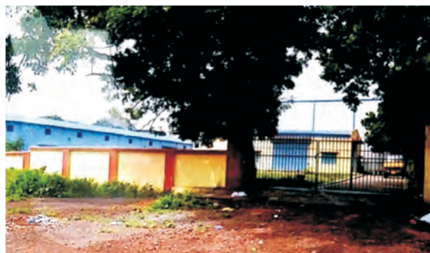
Completion of godown work
