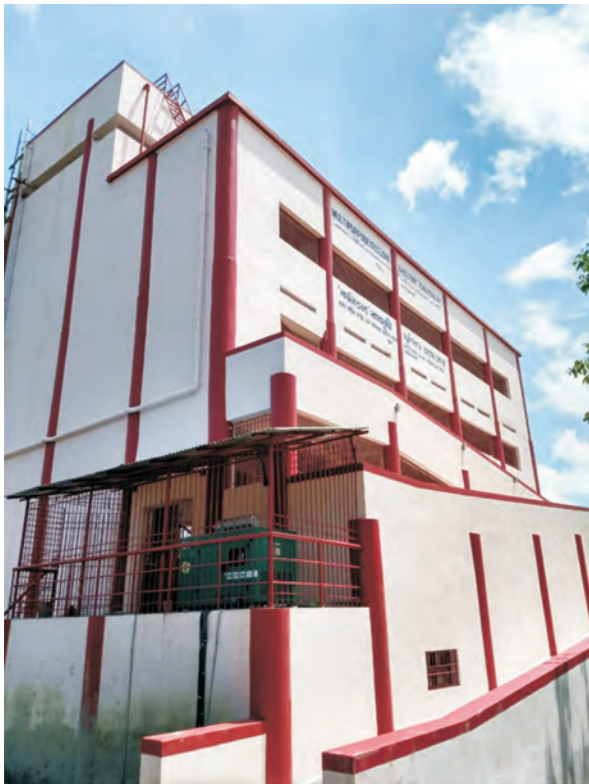
Construction of Cyclone Shelter at Haridashakti in North 24 Parganas District
