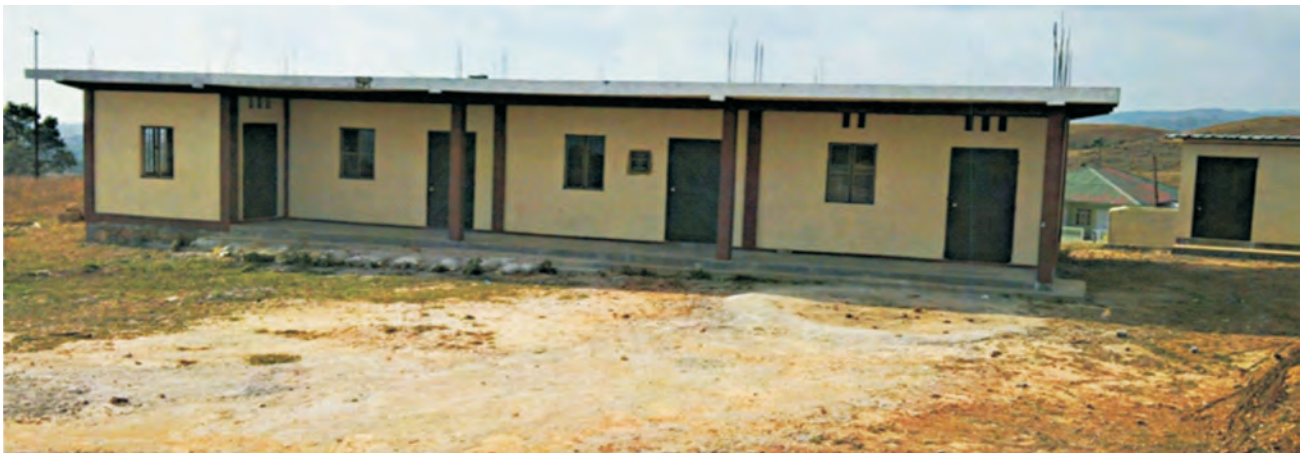
Extension of Lower Primary School at Pynurkba, District East Jaintia Hills (Meghalaya) under BADP, SCA: 2016-17
