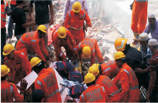
Building collapse at Ghatkopar, near Damodar Park, Lal Bahadur Shastri Marg in Mumbai, MH.
