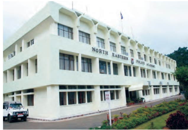
Administrative Building of NEPA
