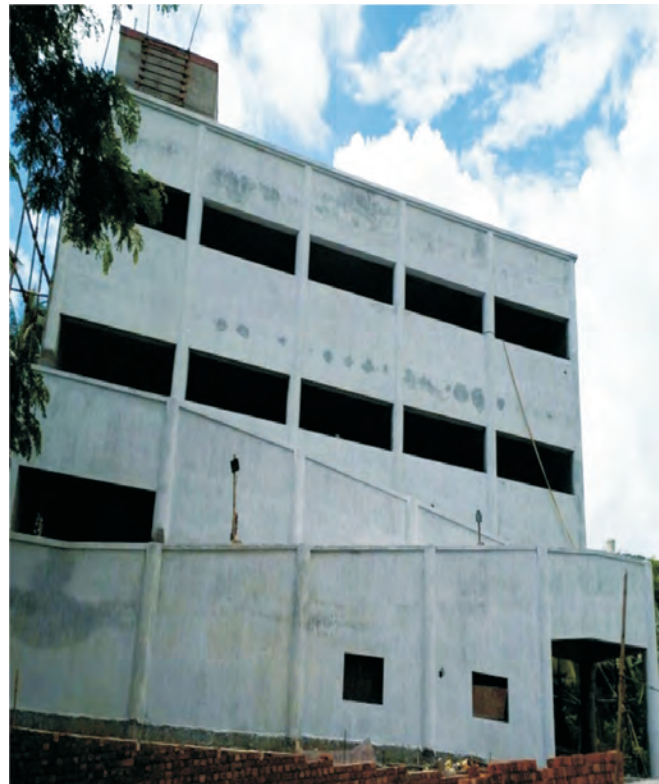
Construction of Cyclone Shelter at Kanya Vidyalaya in East Medinipur District
