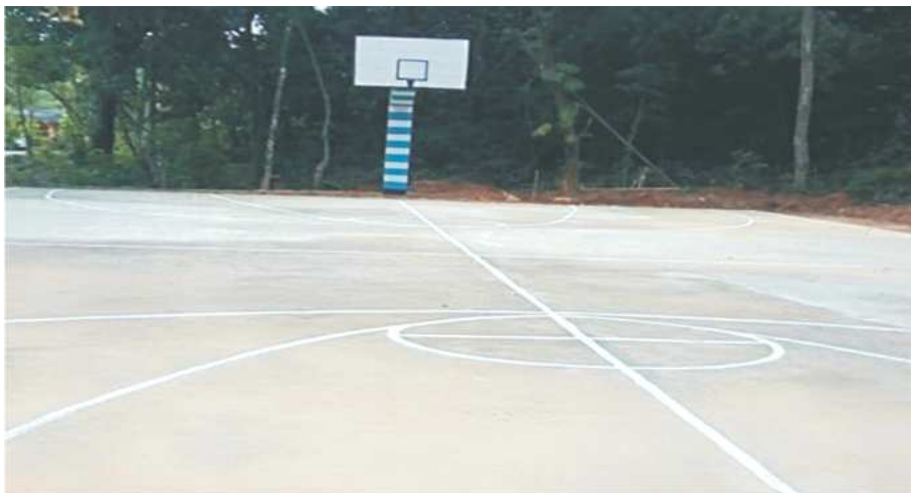
Construction of Basketball Court at Village: Amjalong, Block: Dawki, District: West Jaintia Hills (Meghalaya), Year of Completion: 2019-20
