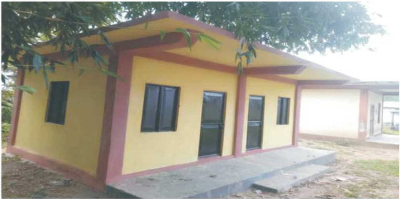
Construction of Additional School Building for Lalpani L. P. School at Village: Lalpani, Block: Mawsynram, District: East Khasi Hills (Meghalaya). Year of Completion: 2019-20
