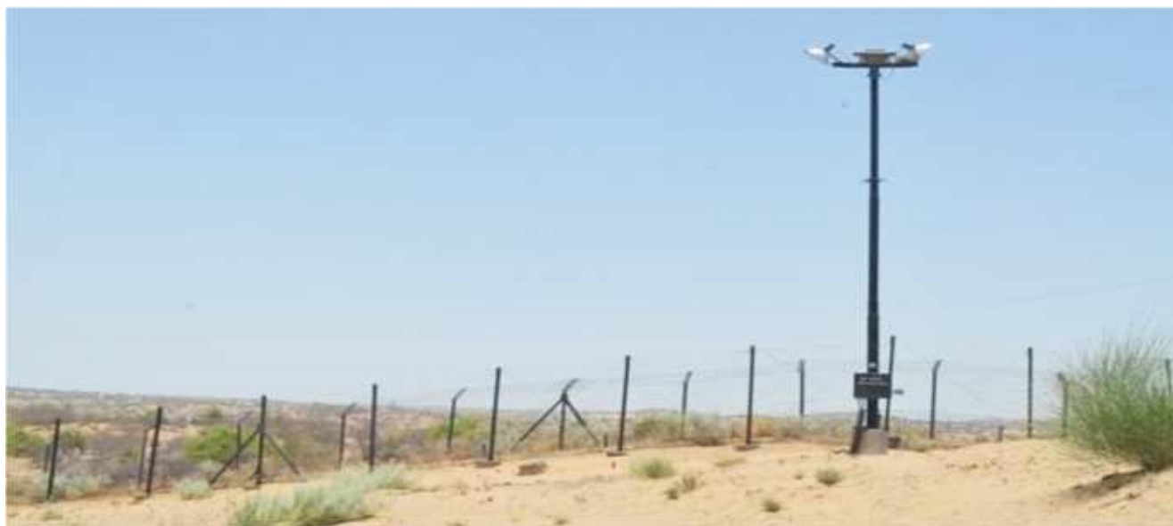
Fence & Floodlighting along Indo-Pakistan Border
