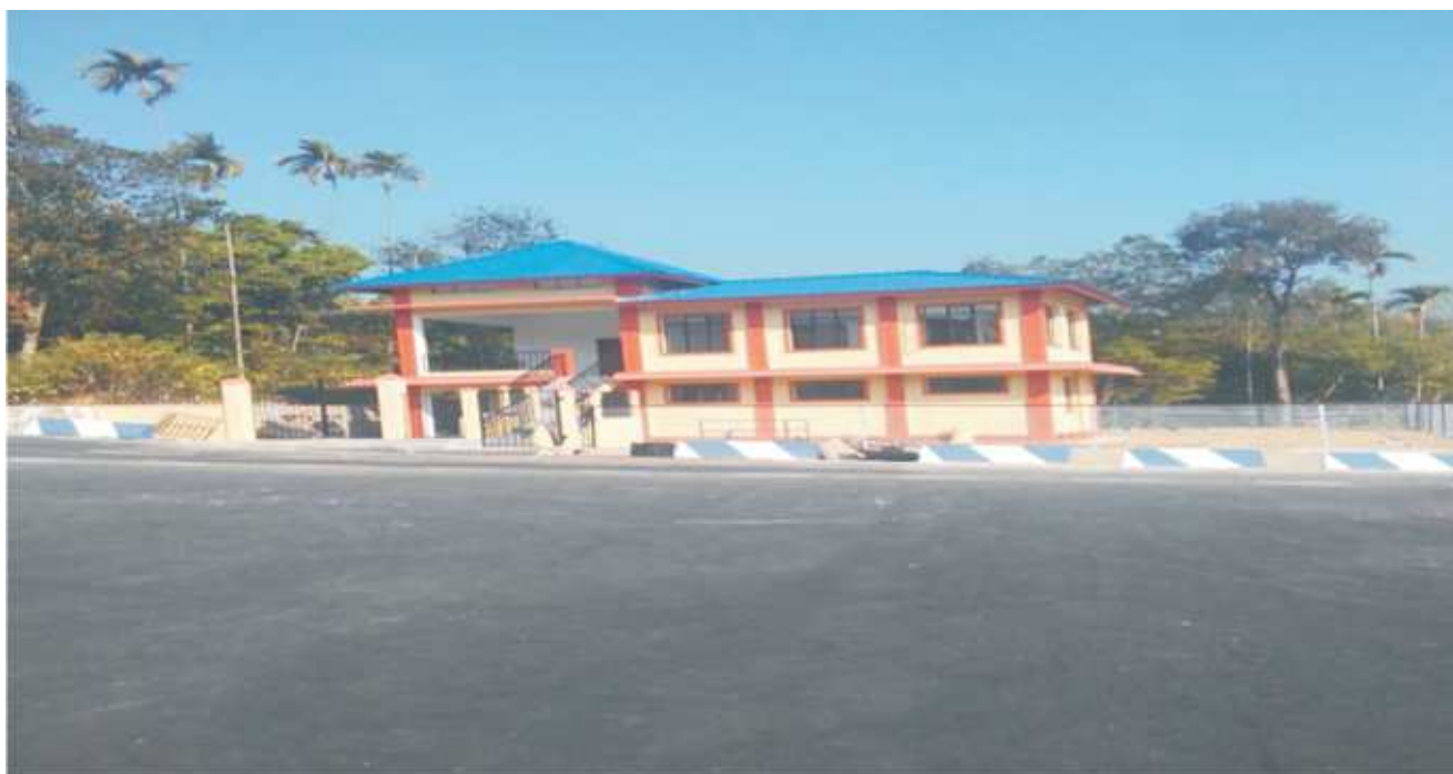
Construction of Tourist Information Centre including electricity and water connection. Village: Mawlynnong, Block: Pynursla, District: East Khasi Hills (Meghalaya). Year of Completion: 2019-20
