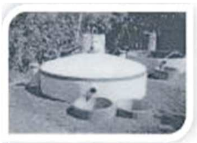
Fixed Dome Deenbandhu Ferro cement Model Biogas Plant (2m 3 ) at Minicoy
