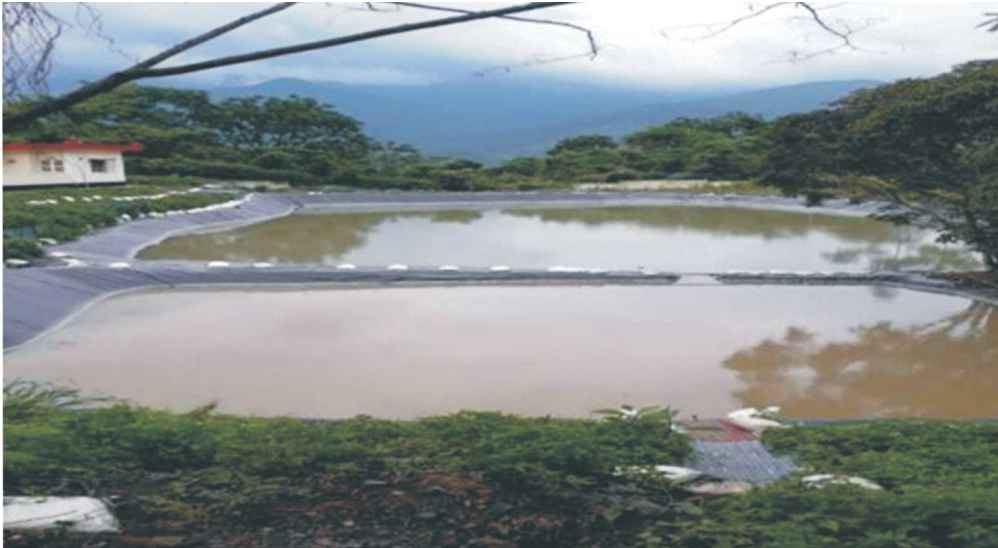
Rain Water Harvesting at Chieswema (Nagaland)
