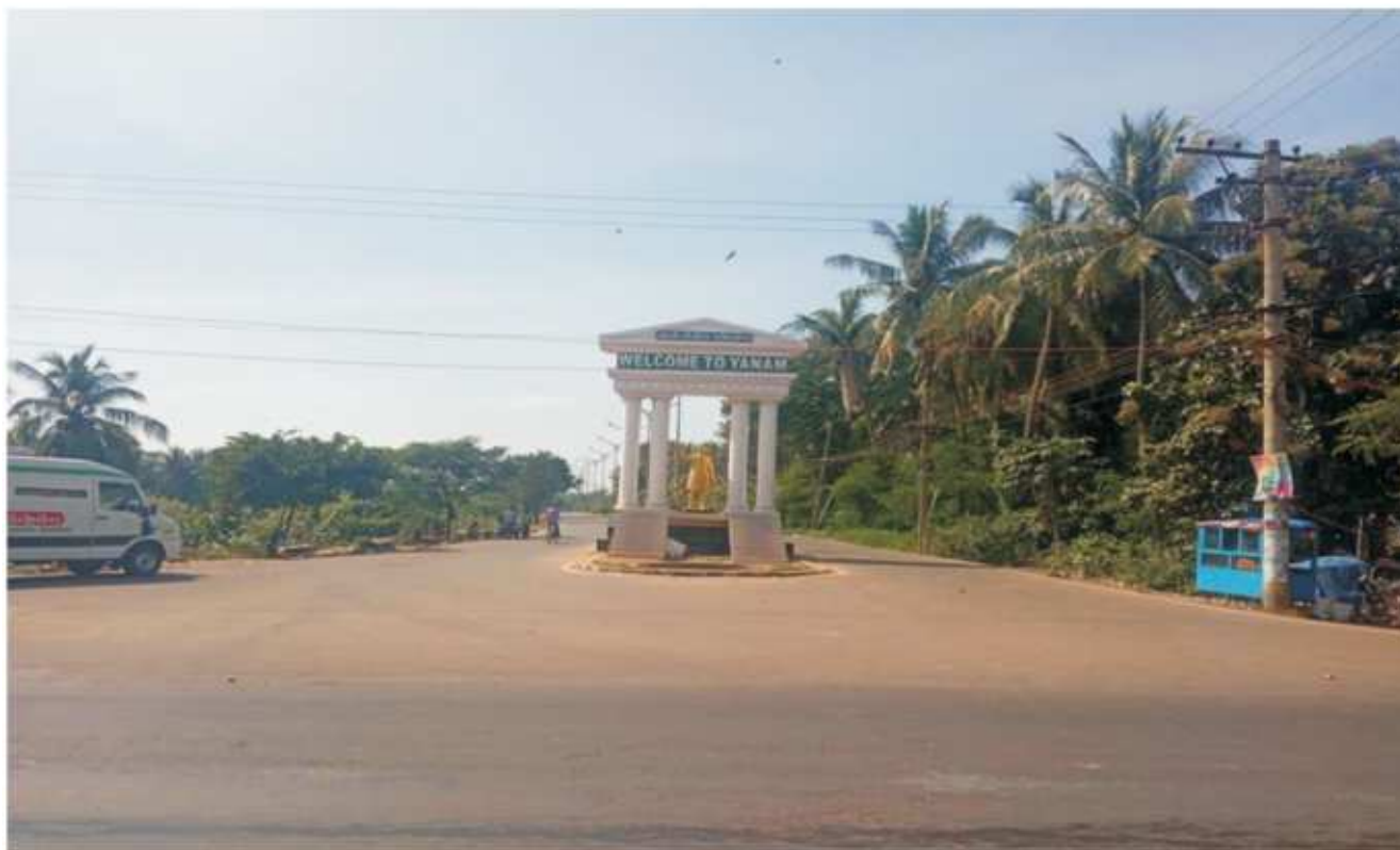
Improvements to the road work taken up at Yanam region
